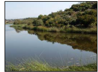
The Dam at Lake Calavera Will Be Fixed
