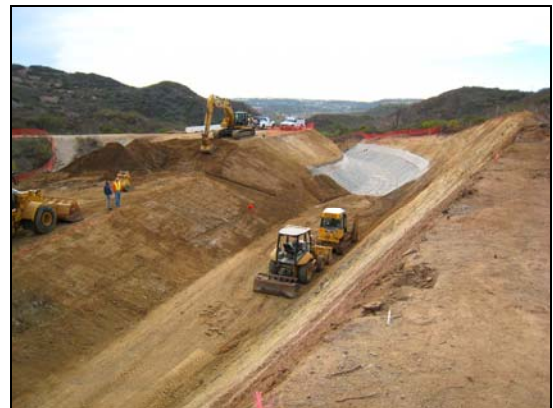
The Calavera Lake Dam 'Spillway' being prepared for concrete.
