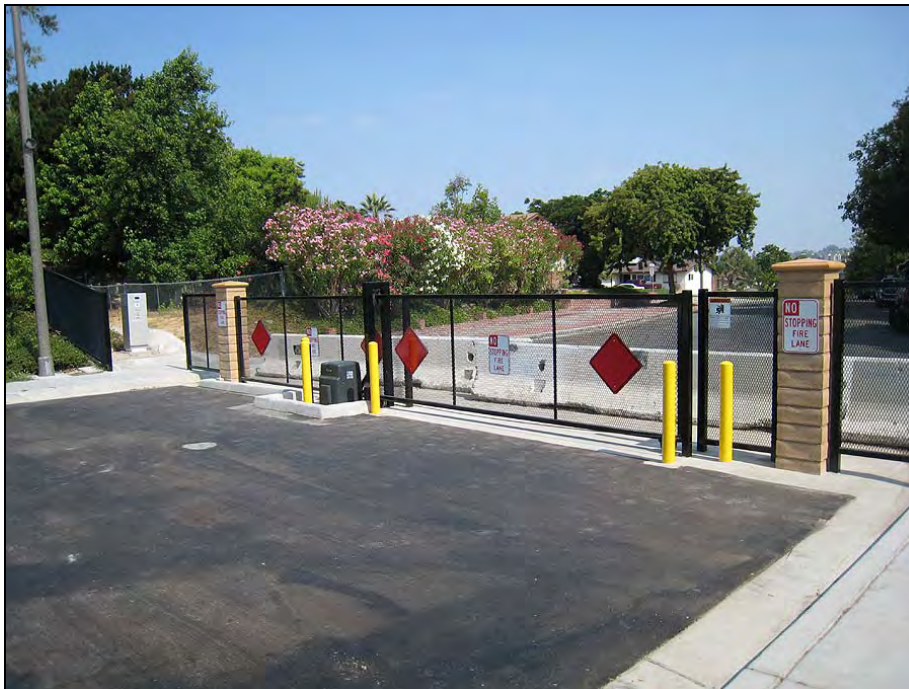
The new gate on Mira Monte Dr, just north of Foothill Ave in Nantucket. The right side slides open when activated by the emergency vehicle activation system.
