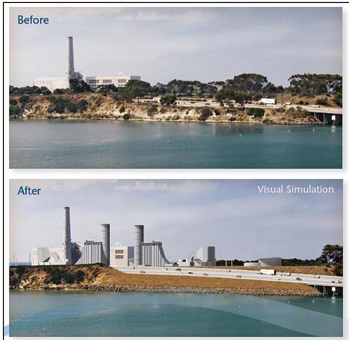
This photo shows the current power and a rendering of the proposed power plant.
