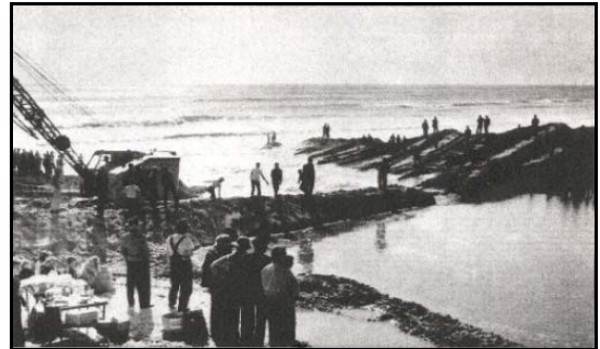
Work on dredging Agua Hedionda Lagoon – mid-20 th century
