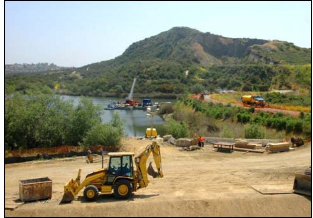
Work continued until late in 2008 on the dam improvements
